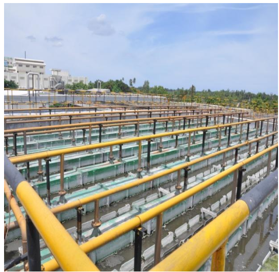
UASBR installed in M/s. Pioneer Jellice India Limited
