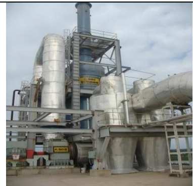
Multi cyclone and Venturi scrubber
