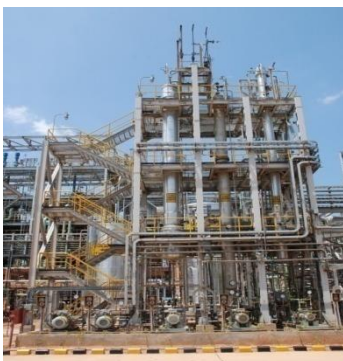
Vent gas absorption system
