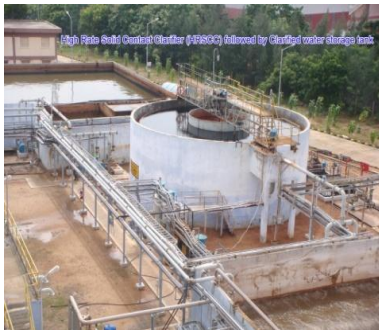
Effluent Treatment plant
