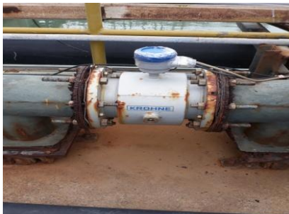
Desalination Reject flow meter
