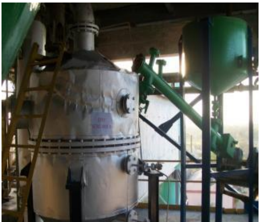
Dry Scrubber in AIF3 Plant
