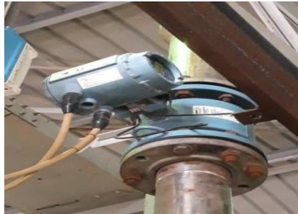
ZLD RO output flow meter
