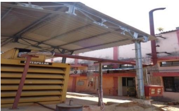
Stack attached to DG set
