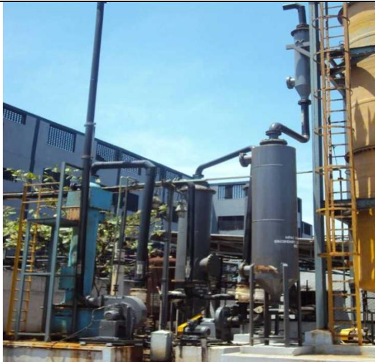
Biofilter replaced with ACF in M/s. Solara Active Pharma Sciences Limited
