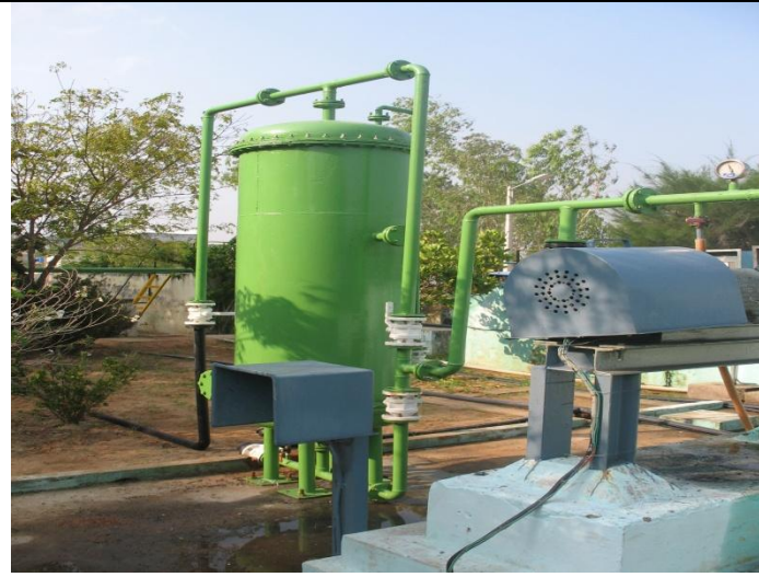
Pressure sand filter installed in M/s. Arkema Peroxide
