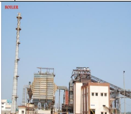
ESP and Stack of Boiler
