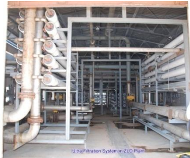
Ultra filtration and RO system
