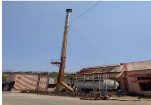
Stack attached to Thermopac
